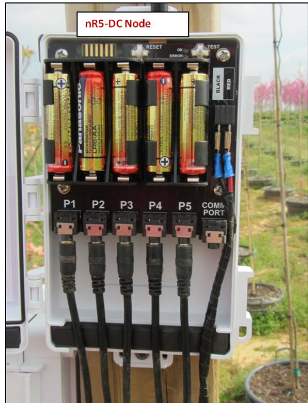
Fig. 56b. The nR5 monitoring and control node, which provides local setpoint (sensor-based) control, in tandem with the 12V-DC latching solenoid (see Fig.4).
