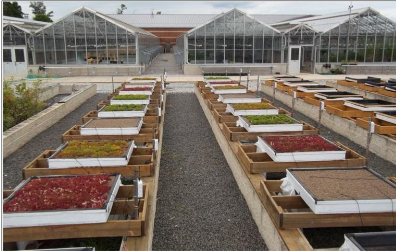
Fig. 62. Green Roof Research Site University of Maryland, Spring 2012
