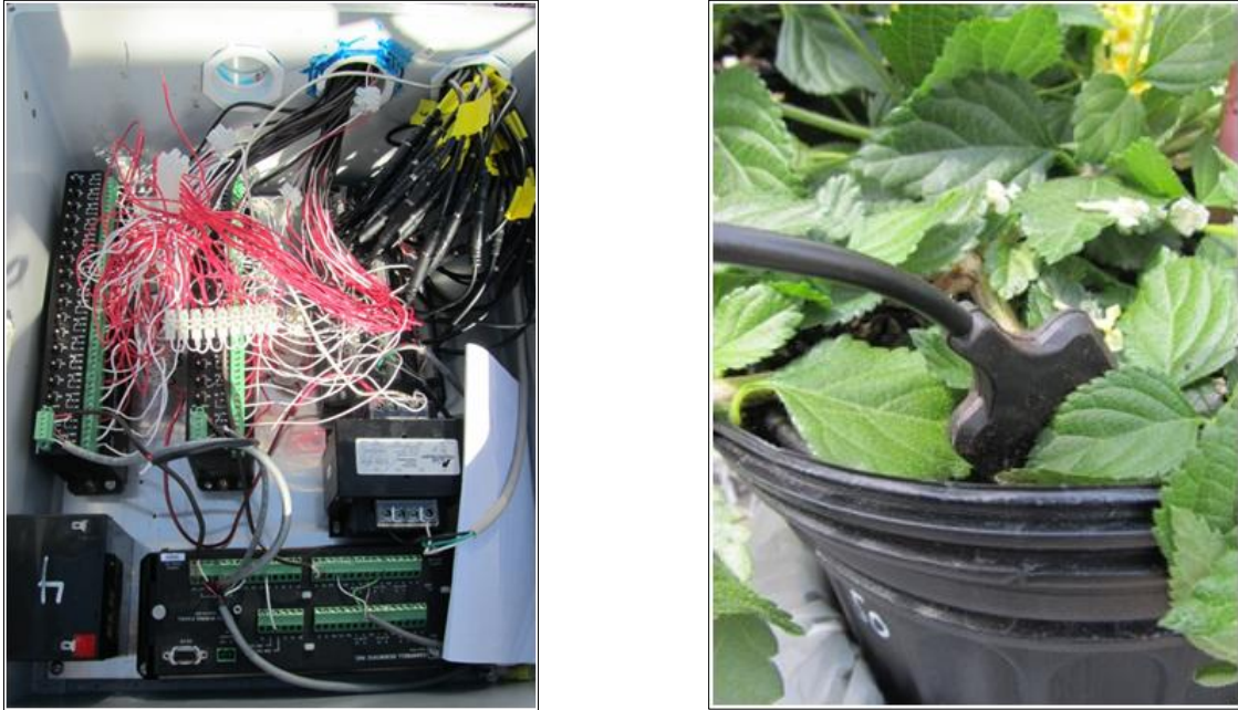
Fig. 39. The wired irrigation control system, with soil moisture sensors connected to a Campbell Scientific multiplexer and 32 solenoids connected to two relay drivers. A CR10 datalogger collects all data and decides when to irrigate the various plots.
